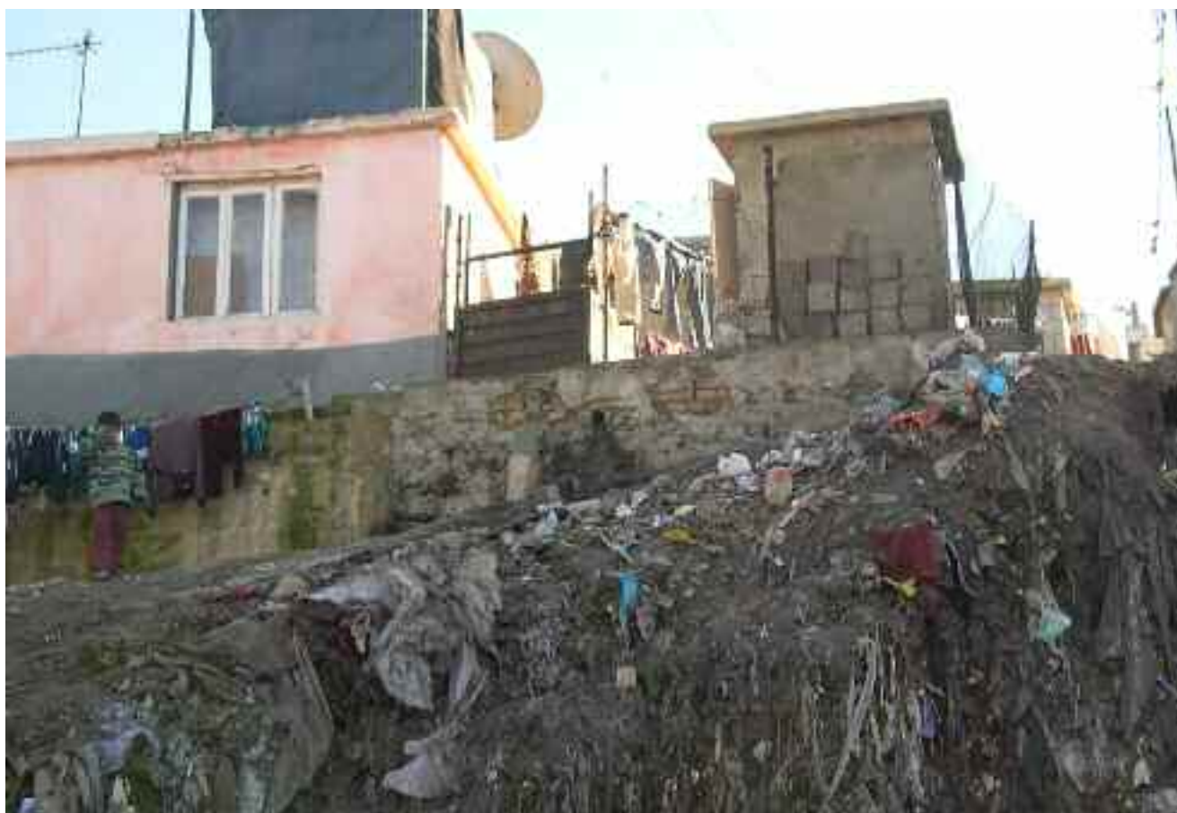
Photo 1: Rubbish dump and a broken sewage pipe around Roma homes.
