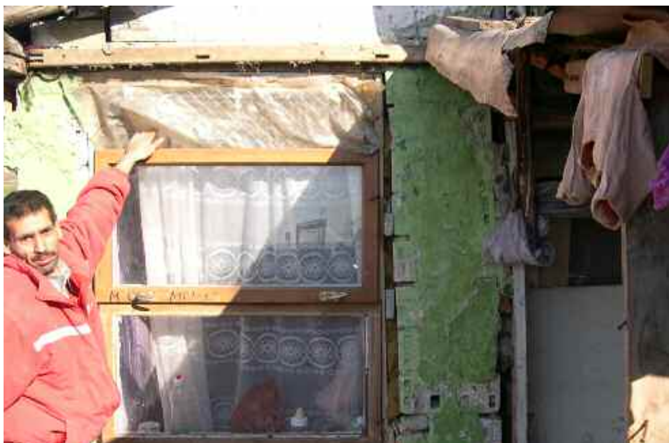
Photo 4: A hole in the wall of Mehmet's shack that he tries to cover with pieces of plastic.
